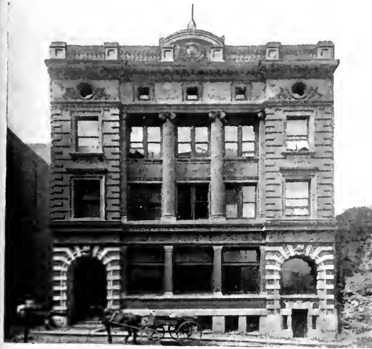
FIG. 1.—MAIN EXCHANGE BUILDING, KANSAS CITY, MO.
